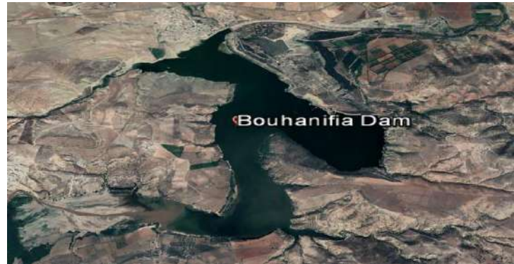
Figure. 1 Aerial view of Bouhanifia dam
